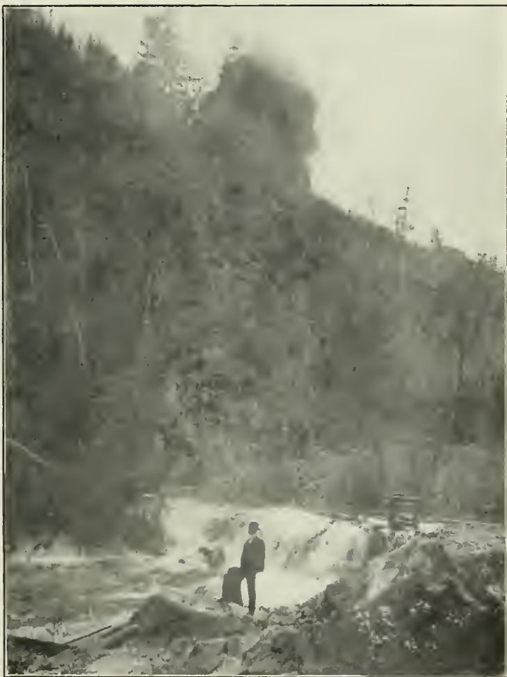
Head gates Banff Waterworks.
