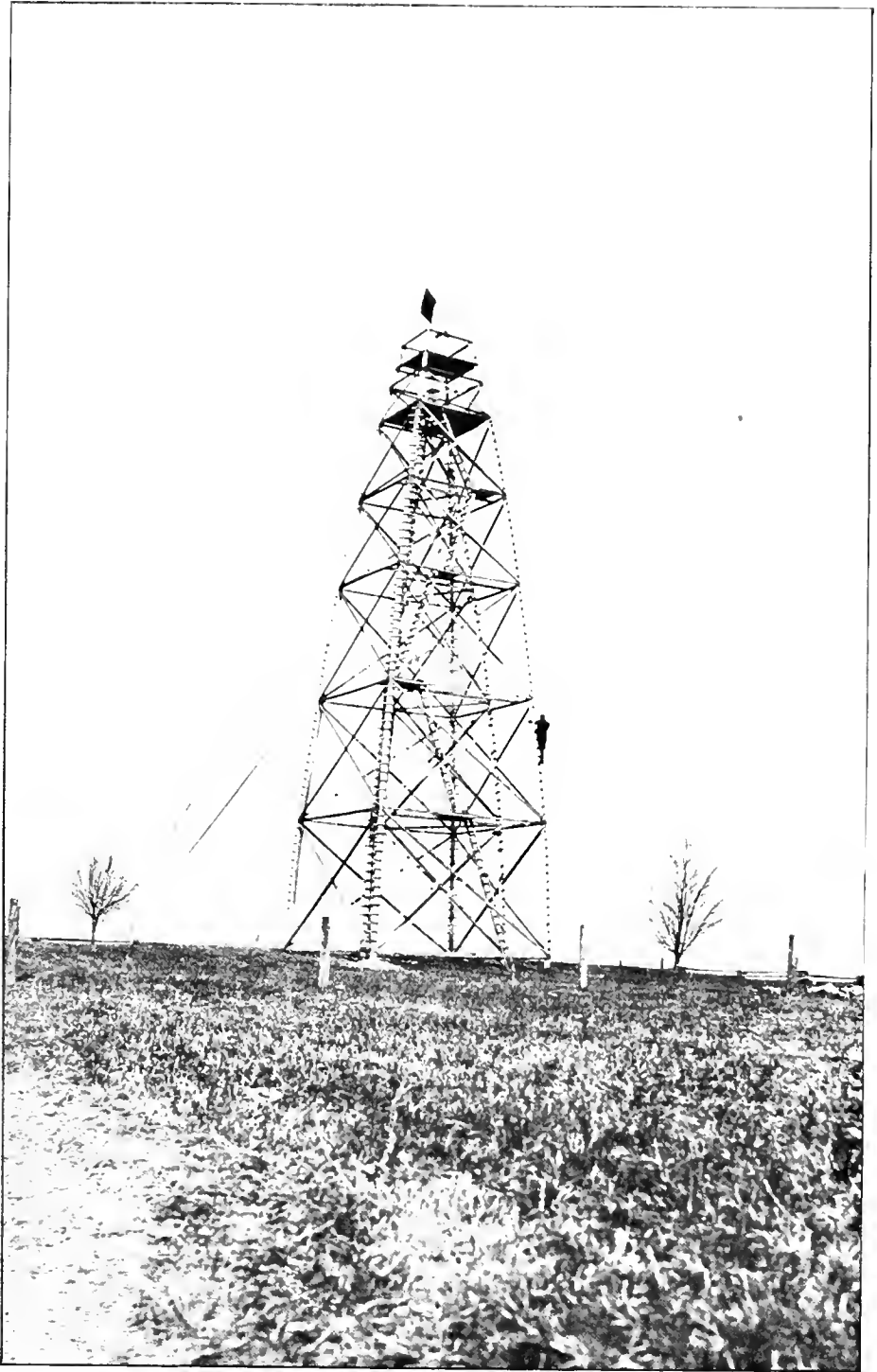
FIG. 2—Observing Tower, eighty-seven feet high, near Bowesville.
