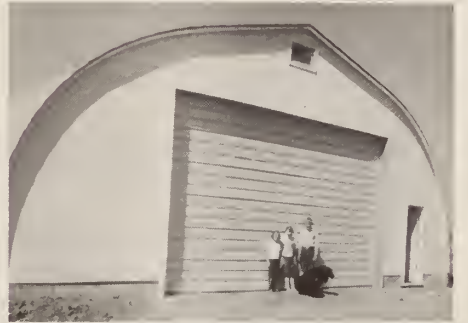
Arch Rib building.
