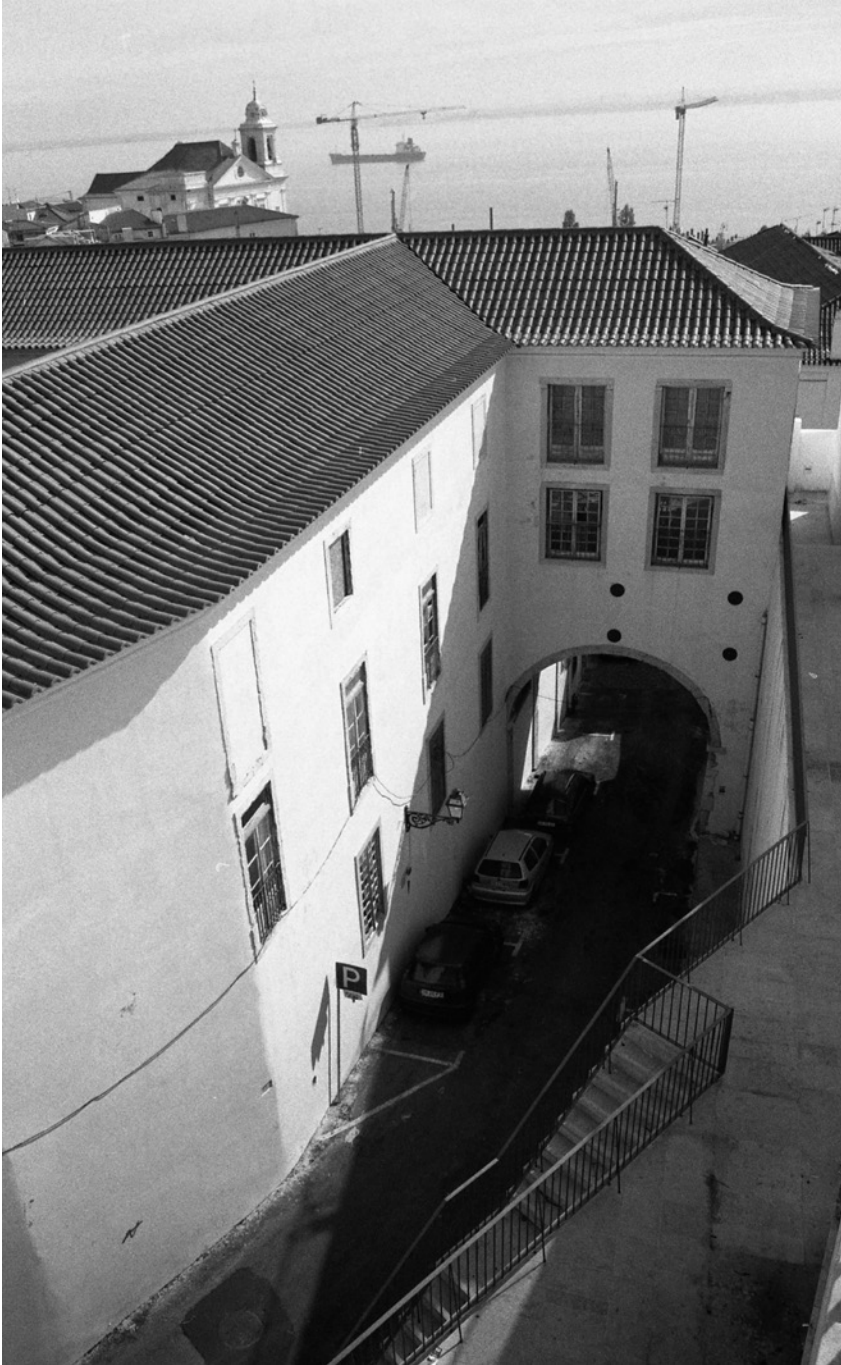
FIGURE 6.4 Current view of the Rua do Salvador in Lisbon, which ended at the church of the Salvador. Photo © Susana Bastos Mateus.
