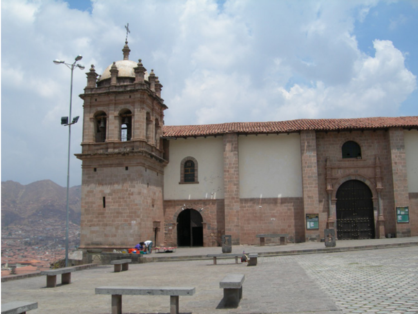
FIGURE 3.6 San Pedro, in Cuzco, formerly Nuestra Señora de los Remedios or Parish of the Hospital de Naturales. Although the church stands in the place where it was founded, this temple was built in the seventeenth century, most likely after the 1650 earthquake. Photo © Gabriela Ramos.
