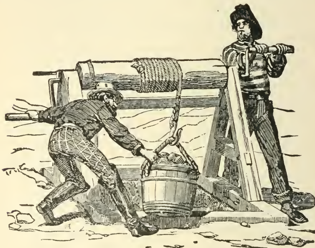
MINERS SINKING A SHAFT.
