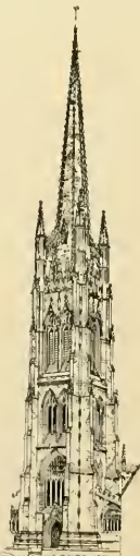
G ST. JAMES LOUTH, Lincs. & ANGLE TURRETS & FLYING BUTTRESSES
